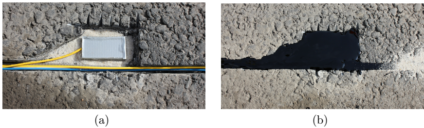
Fig. 3. PDMS-FBG sensor placement in widened milled in groove (a); PDMS-FBG sensor covered with cold asphalt (b).
